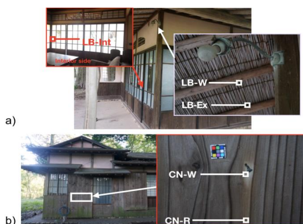
Fig. 2 Investigation point of the Arbor a) investigation points of exterior
